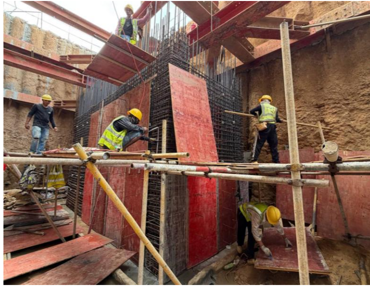
Installation of Formwork of Core Walls
