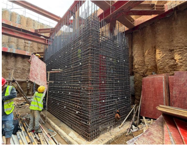
Installation of Rebar of Core Walls
