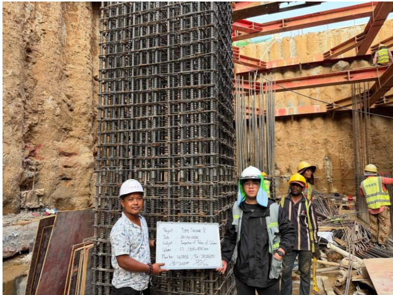
Inspection of stump columns
