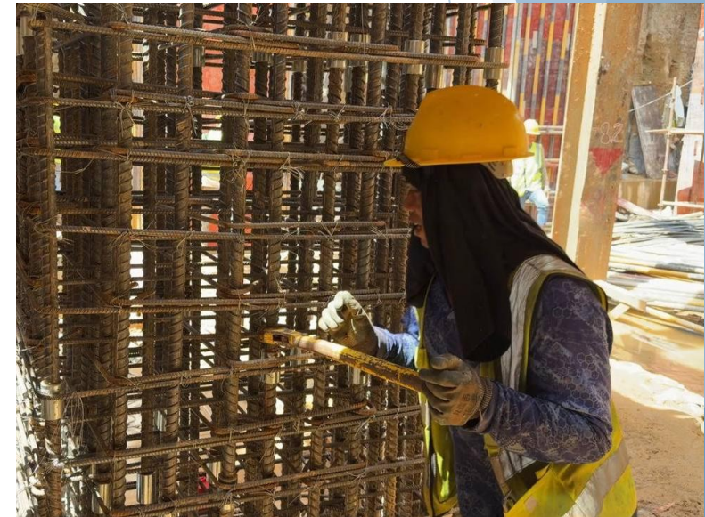
Check coupler tightness
