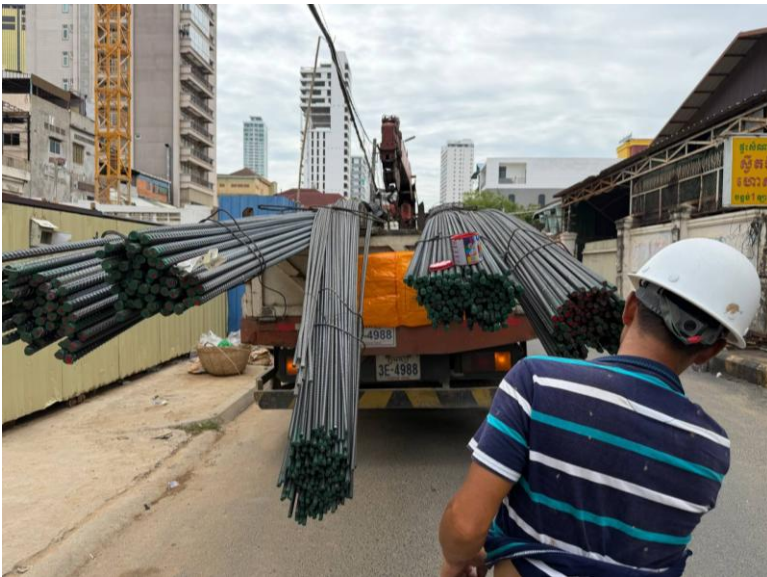
Inspection delivered rebar
