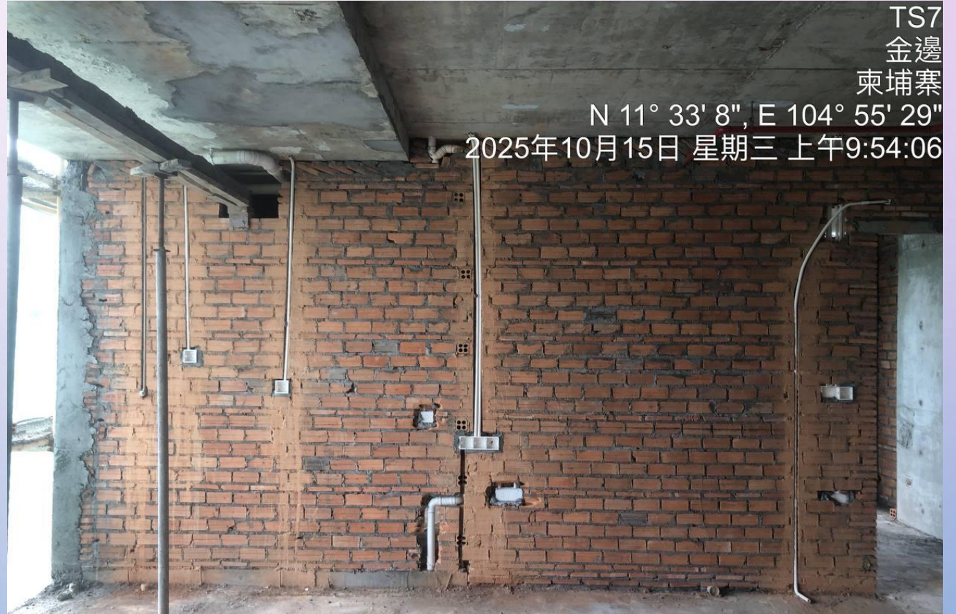
MEP Embedment work
