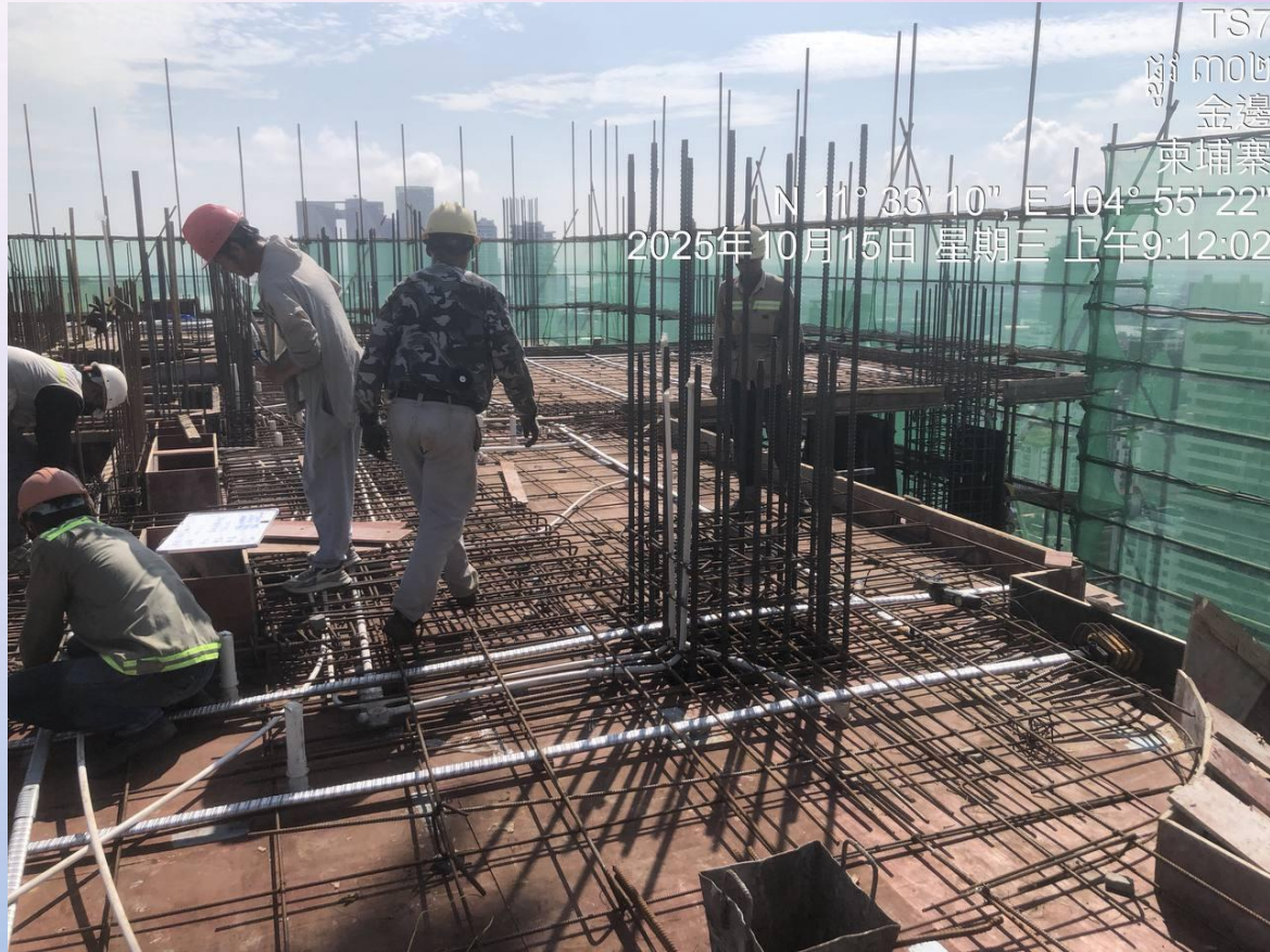
Installation the Rebar of 38MF
