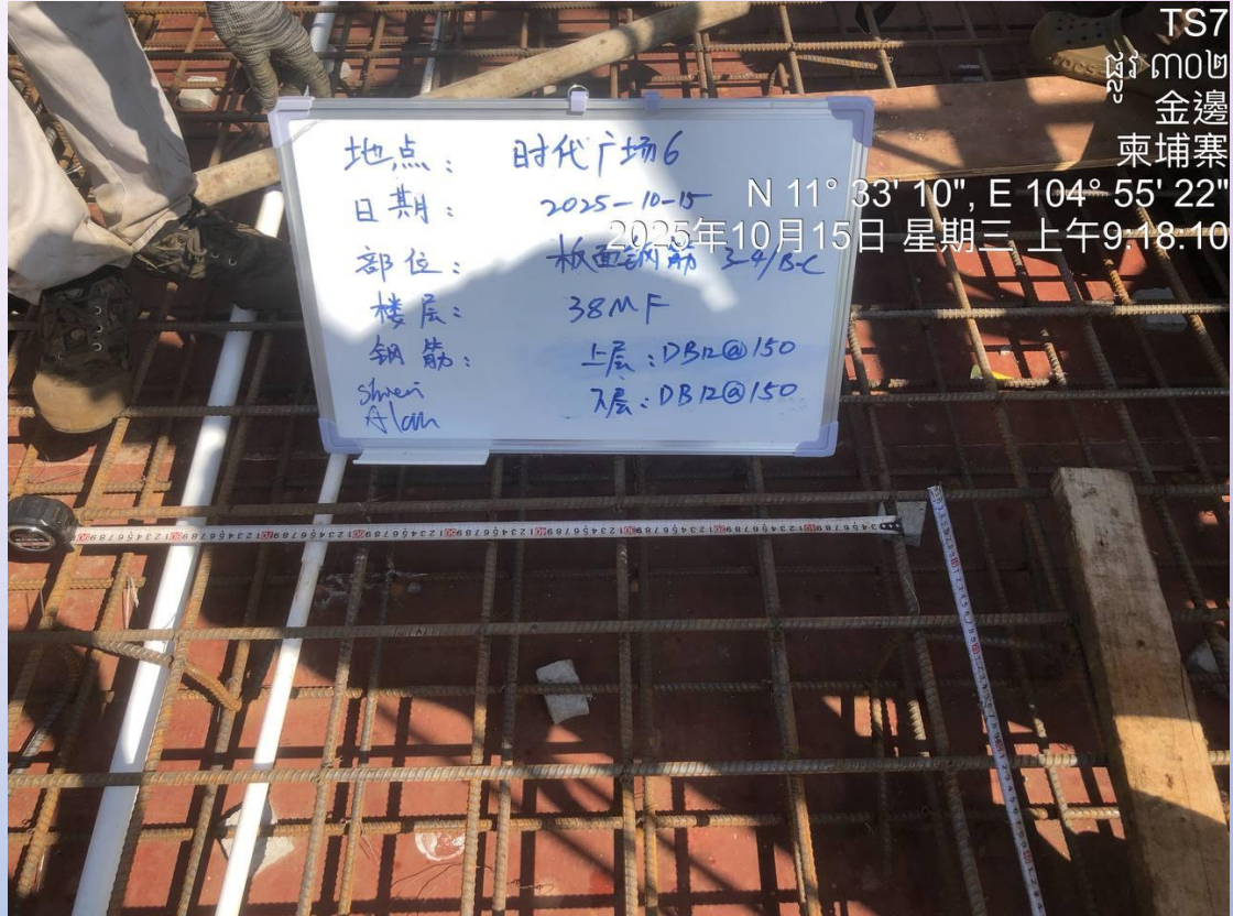
Inspection the Rebar of Slab: 37MF
