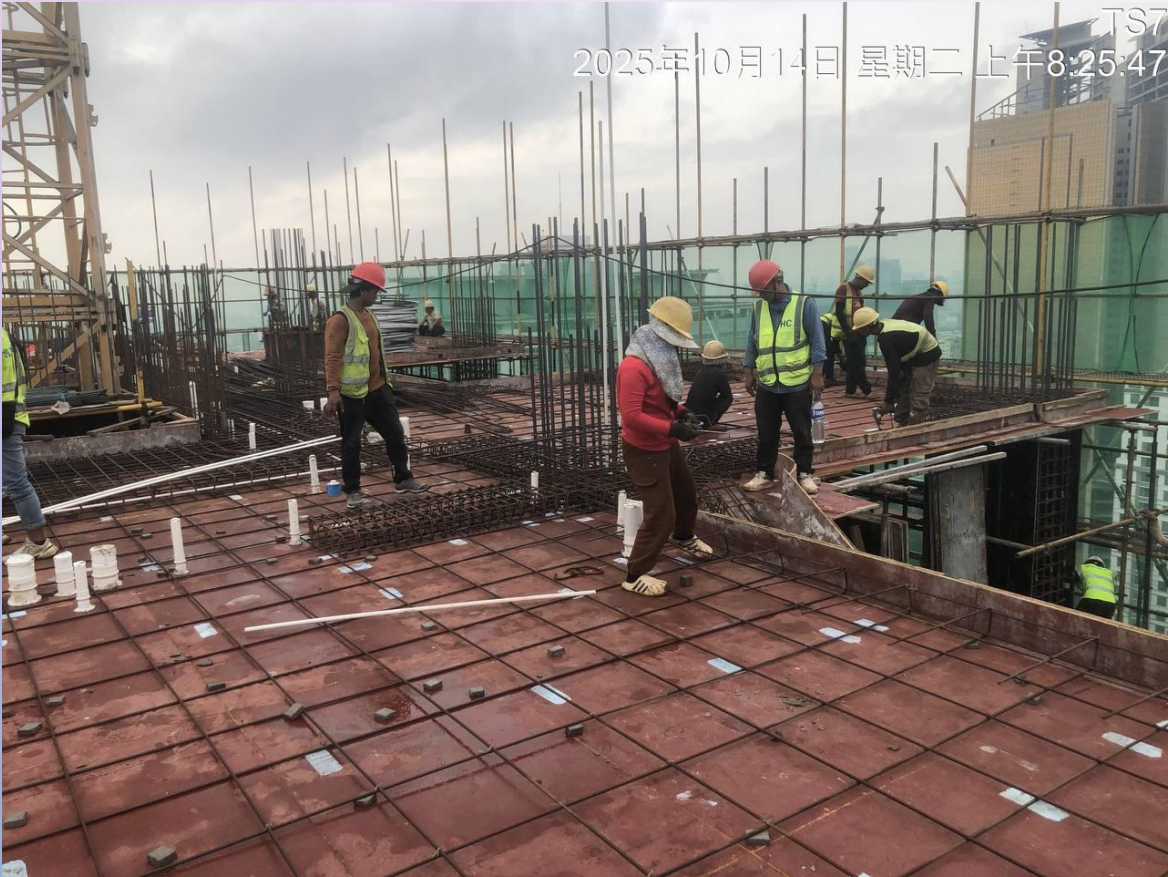
Installation the Rebar of 38MF
