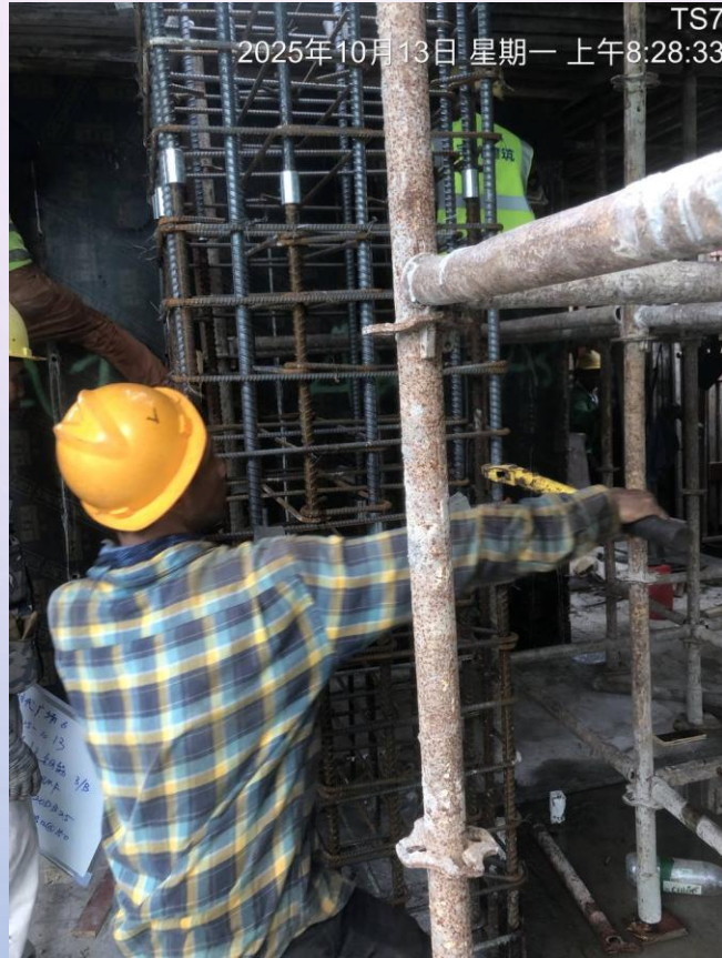
Inspection the rebar of Column & Wall : 38F
