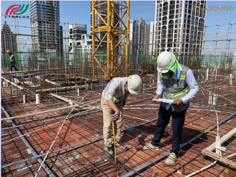
Inspection the PT of Slab: 27F
