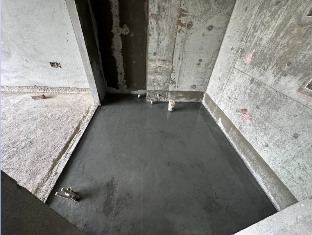
Inspection of Waterproofing work
