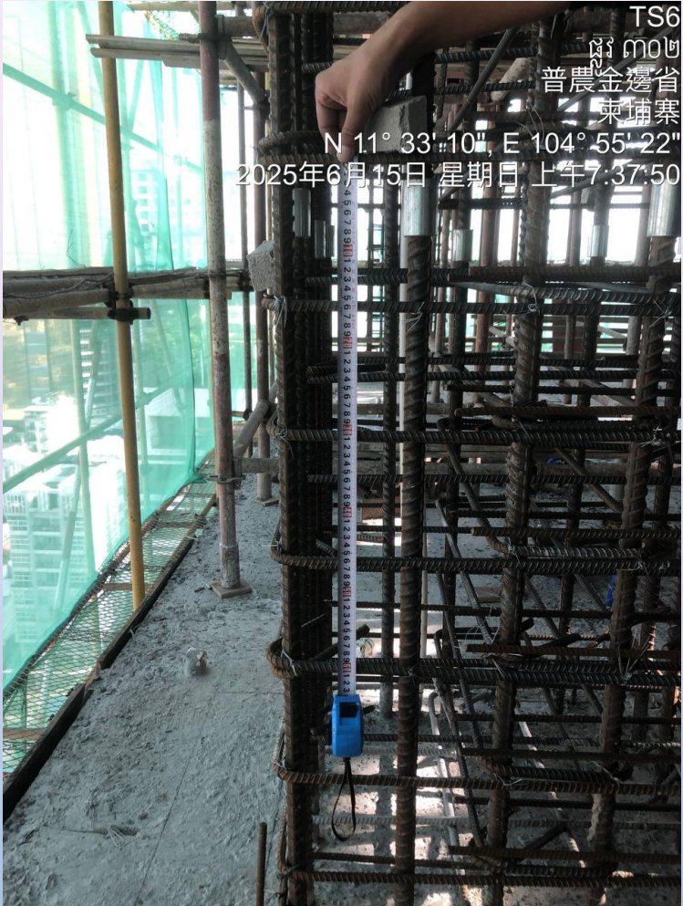
Inspection the rebar of Column & Wall : 26F
