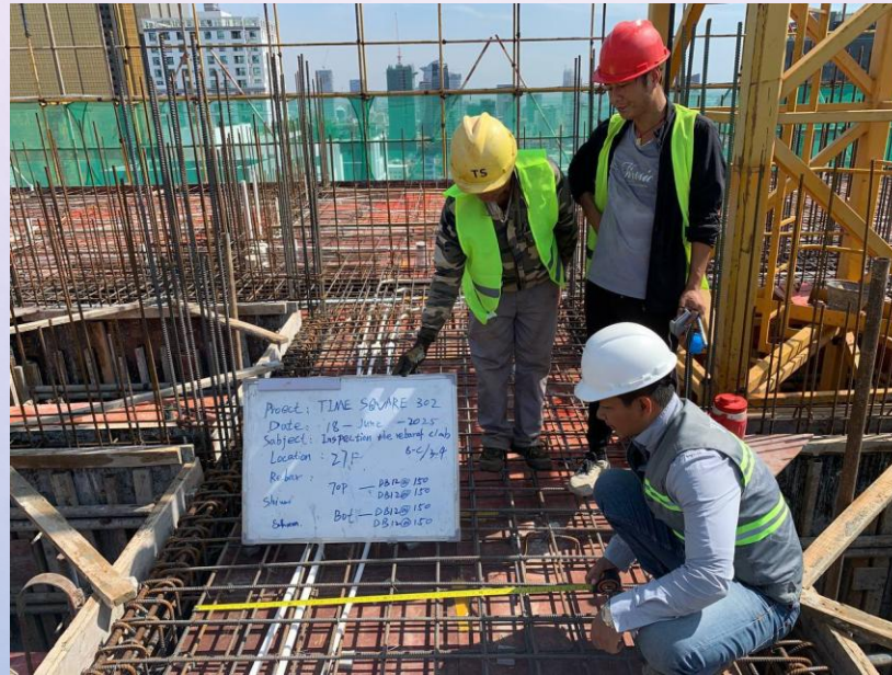
Inspection the Rebar of Slab: 27F
