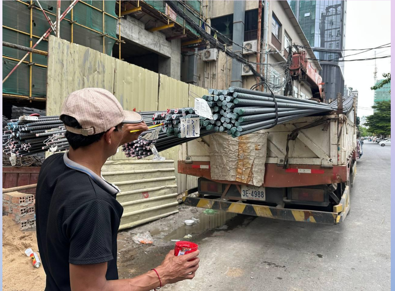
Inspection the rebar
