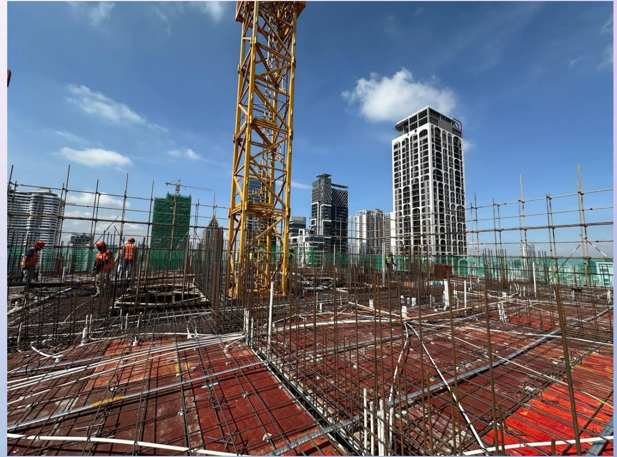
Installation the Rebar of 27F
