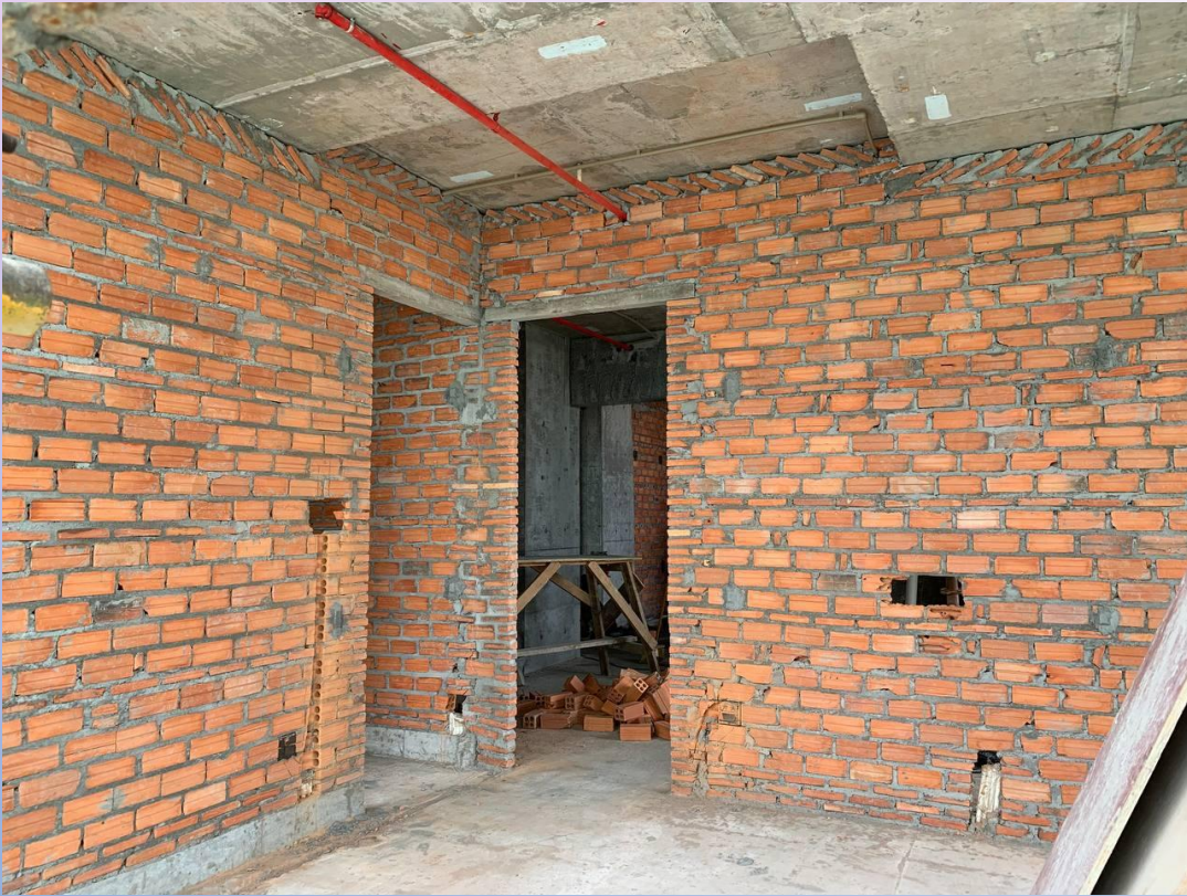
Inspection of brick wall installation work
