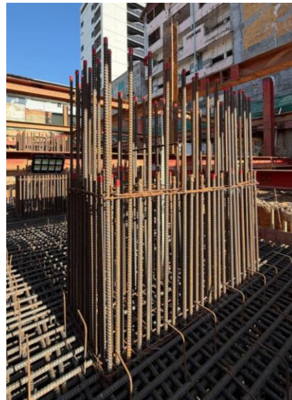
Inspection of starter rebar of columns
