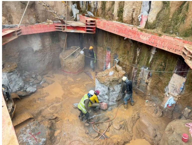
Pile chipping and breaking work
