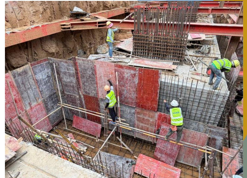
Install formwork of wall
