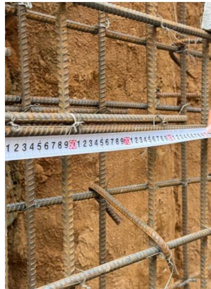
Inspection of rebar of Septic Tank
