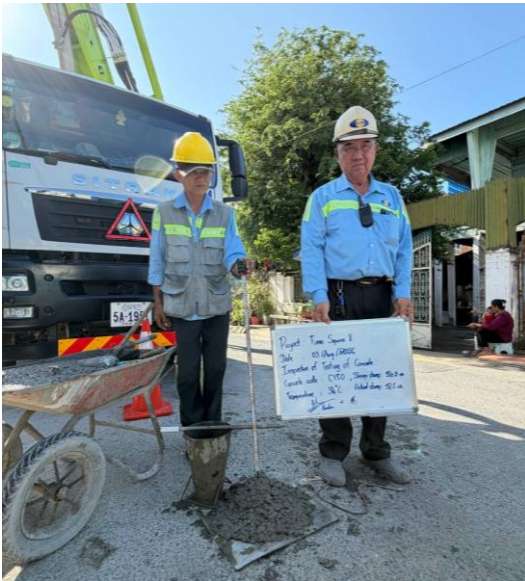
Inspection of concrete
