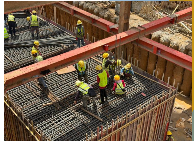
Install starter bars of columns
