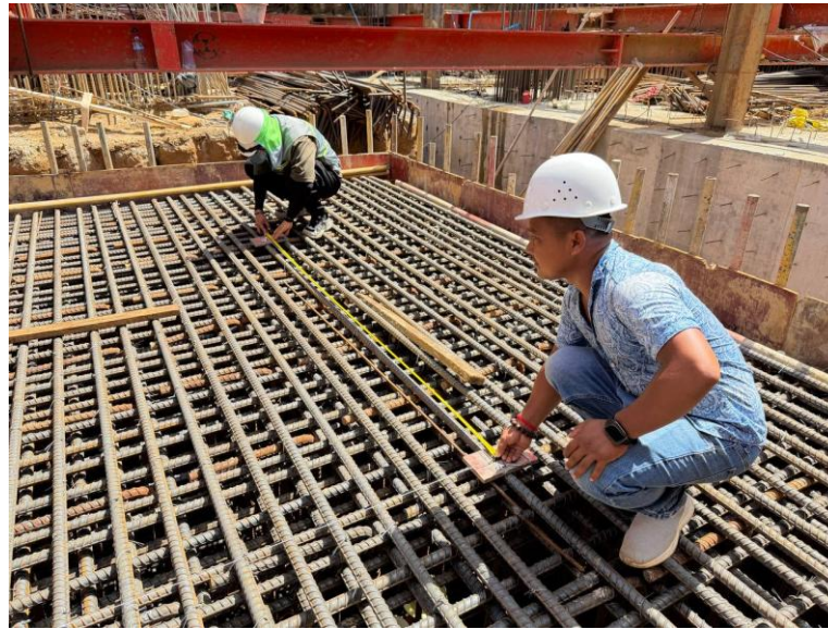
Inspection of Top and Hook bar of PC4
