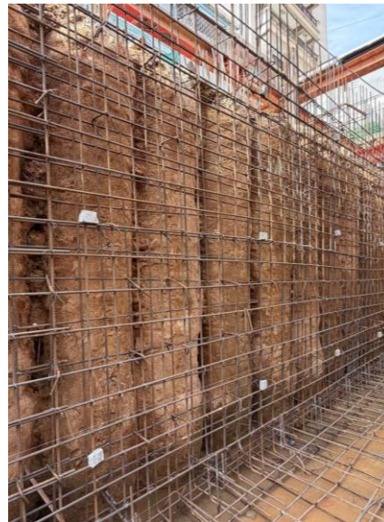
Inspection of rebar of Septic Tank
