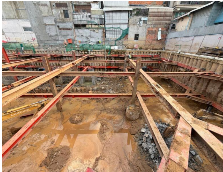
Installation of 2 nd Layer Strut (LVL -4.90M)
