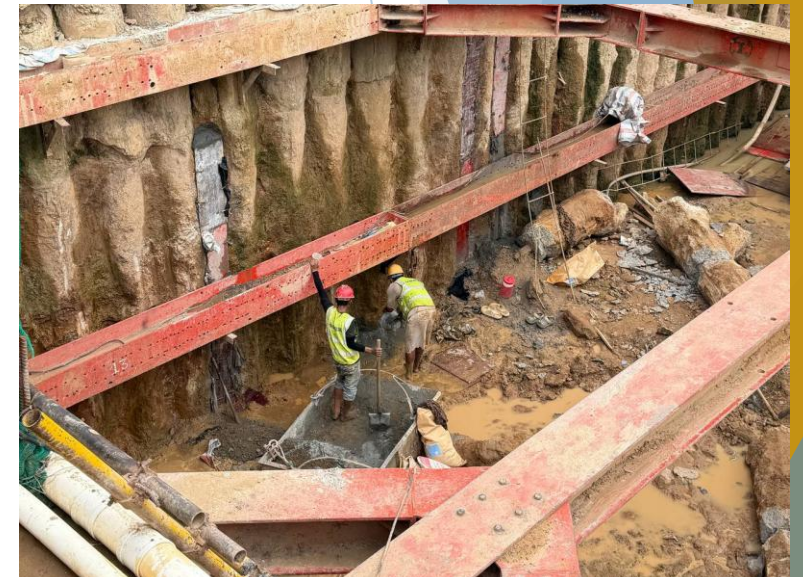
Stop water leaking
