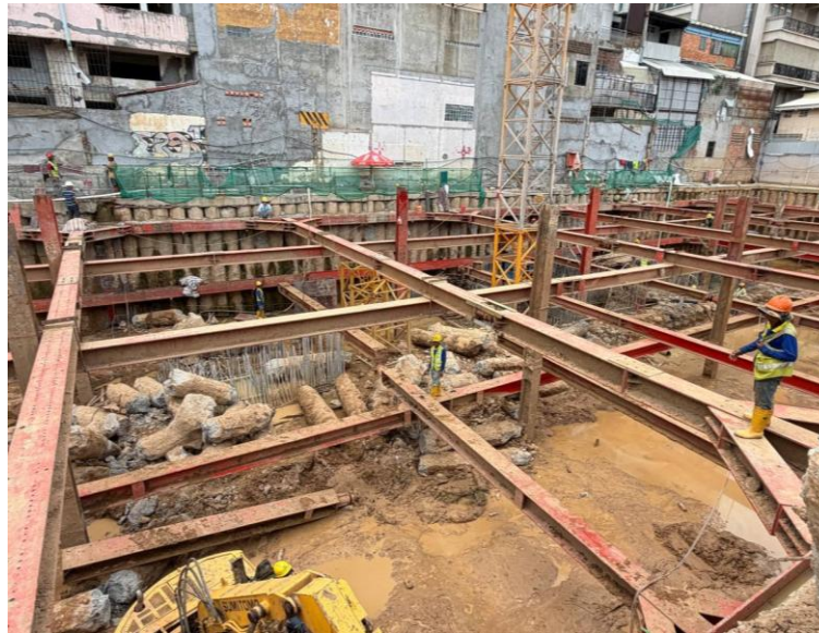
Installation of 2 nd Layer Strut (LVL -4.90M)
