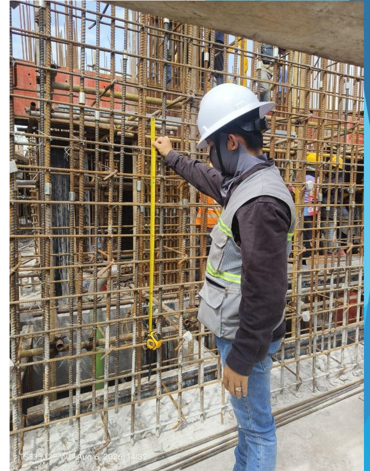
12F Column & Wall Rebar Installation Inspection
