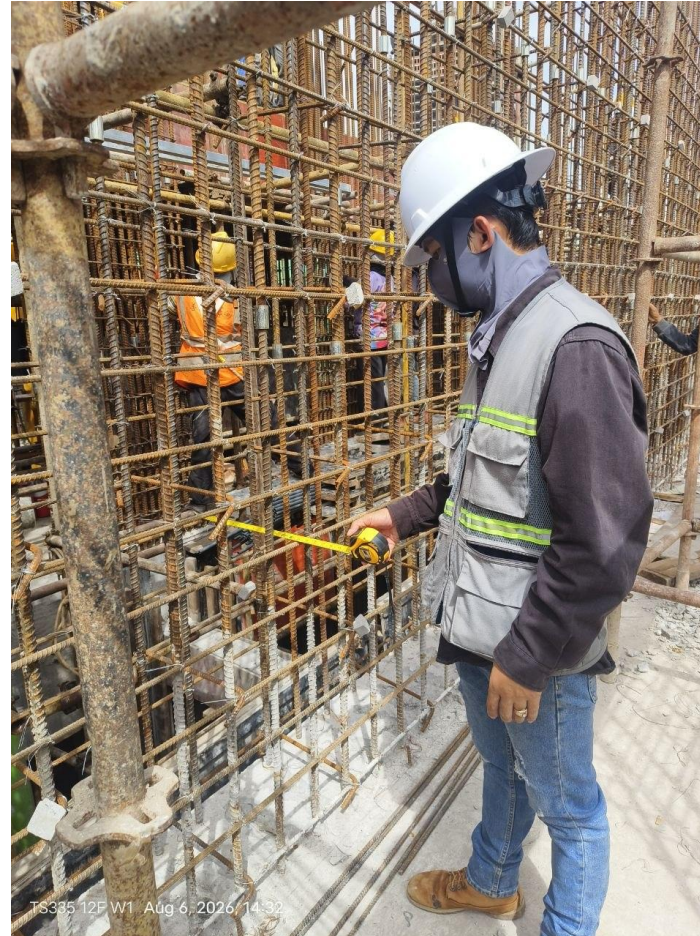
12F Column & Wall Rebar Installation Inspection
