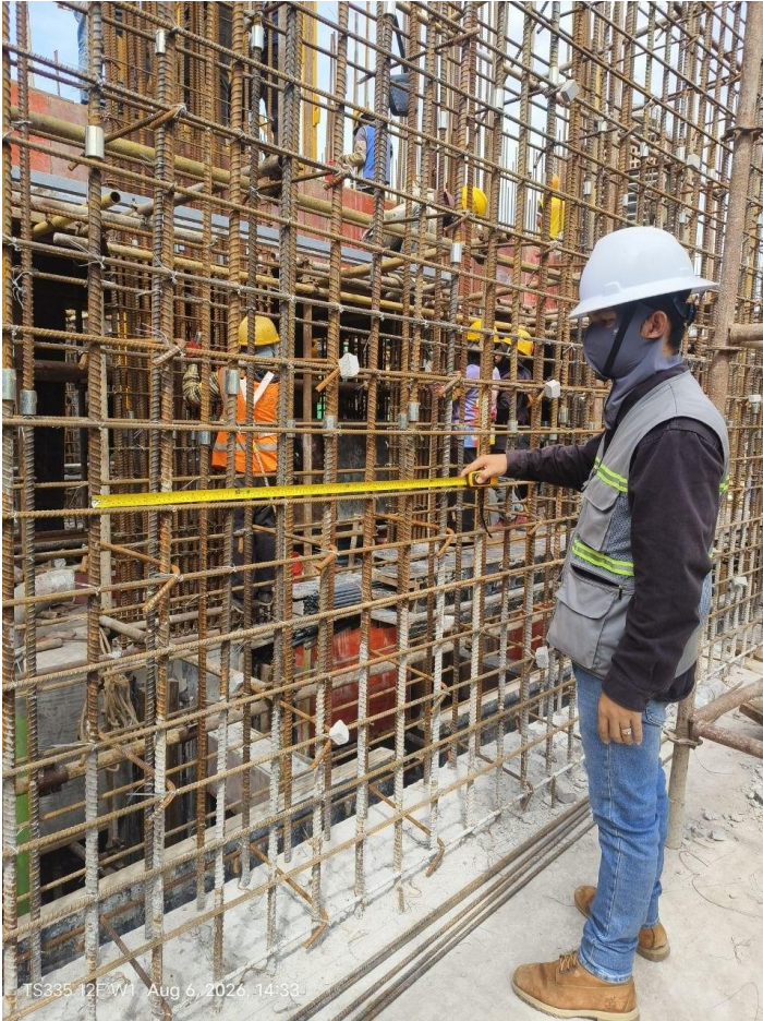
12F Column & Wall Rebar Installation Inspection
