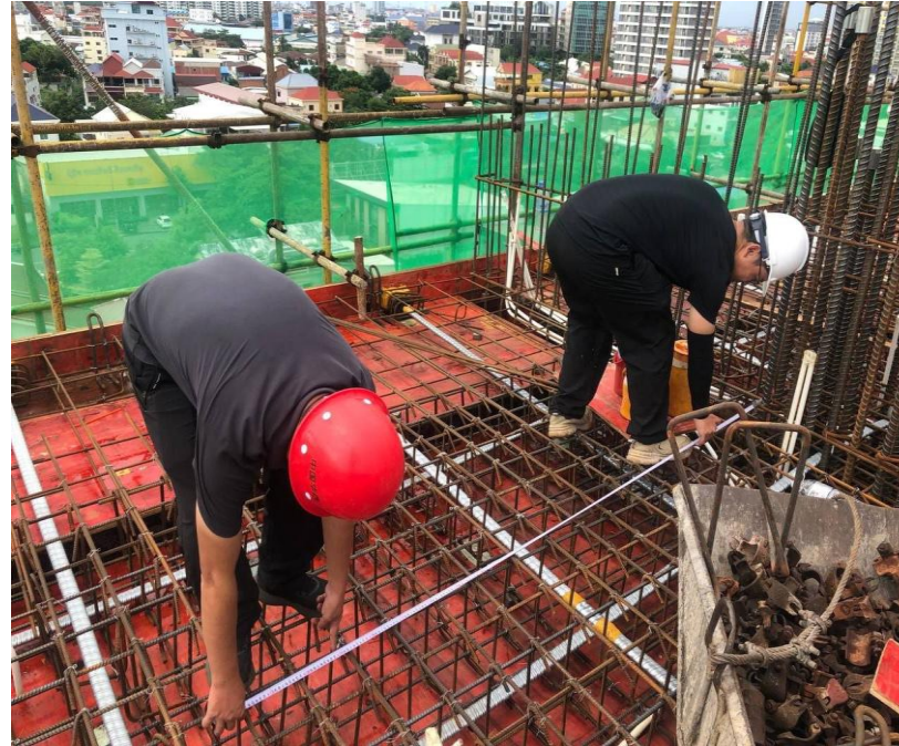
9F MEP Inspection Sleeve & Conduit installation inspection
