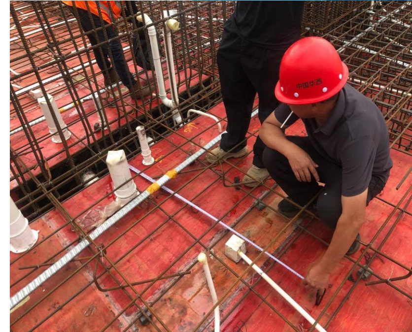
9F MEP Inspection Sleeve & Conduit installation inspection
