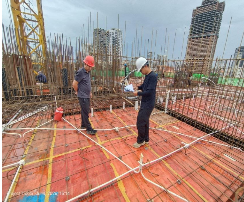
9F MEP Inspection Sleeve & Conduit installation inspection
