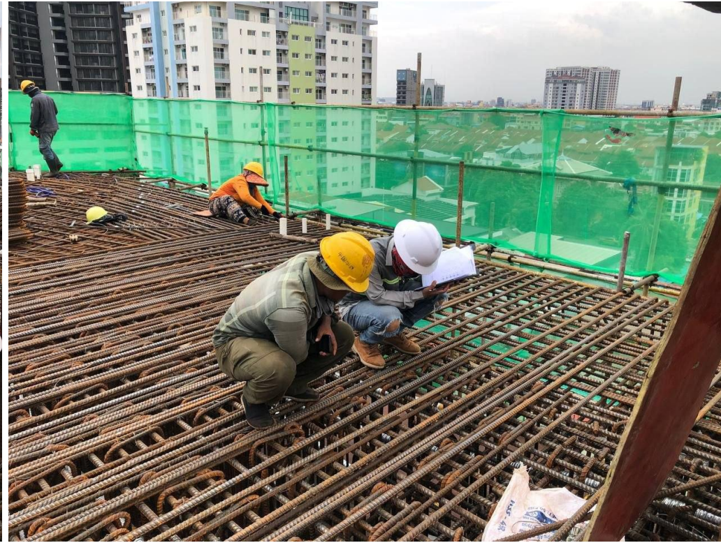
8F Beam Rebar Inspection
