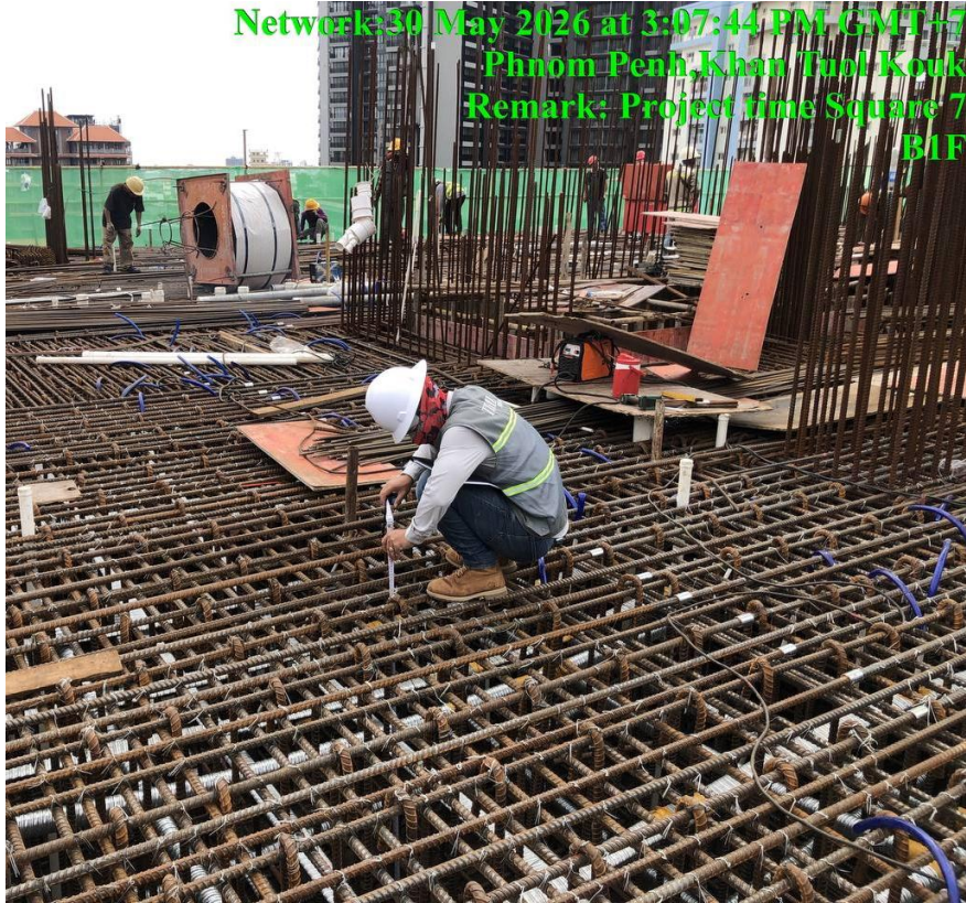
8F Slab Rebar Inspection
