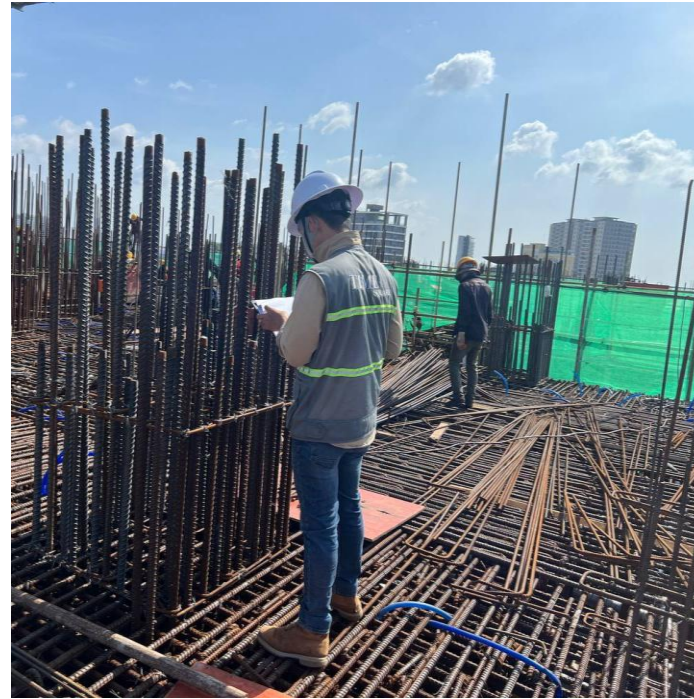
8F Column & RC wall Rebar Inspection
