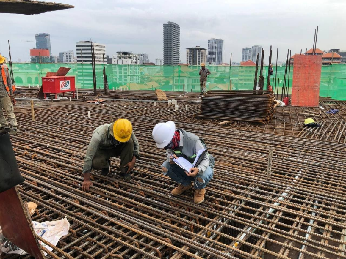
8F Beam Rebar Inspection
