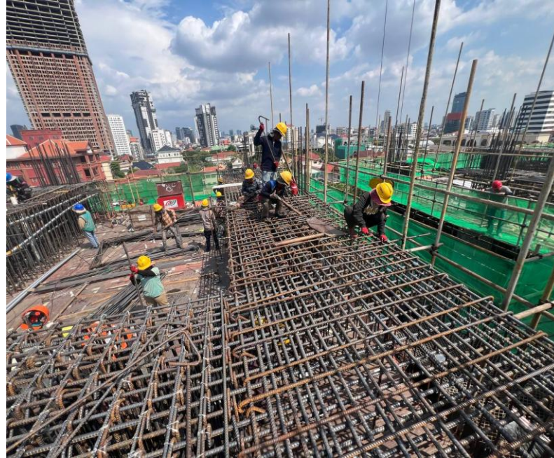
8F Beam Rebar installation
