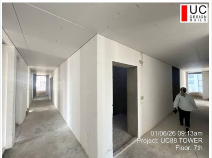
Floor: 7F Date: 06-Jan-2026 Work: Skim coat work
