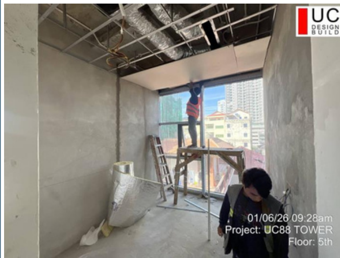
Floor: 5F Date: 06-Jan-2026 Work: Ceiling work
