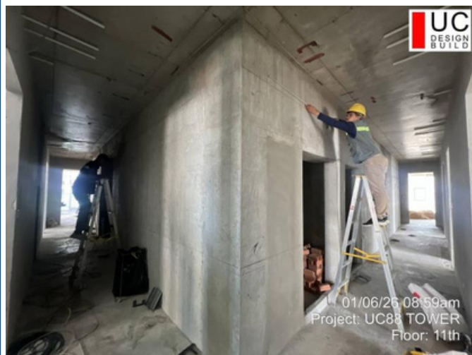
Floor: 11F Date: 06-Jan-2026 Work: MEP work
