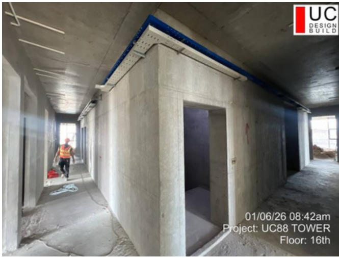
Floor: 16F Date: 06-Jan-2026 Work: MEP work
