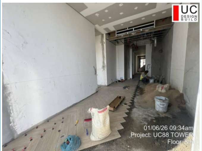
Floor: 5F Date: 06-Jan-2026 Work: Tiling work
