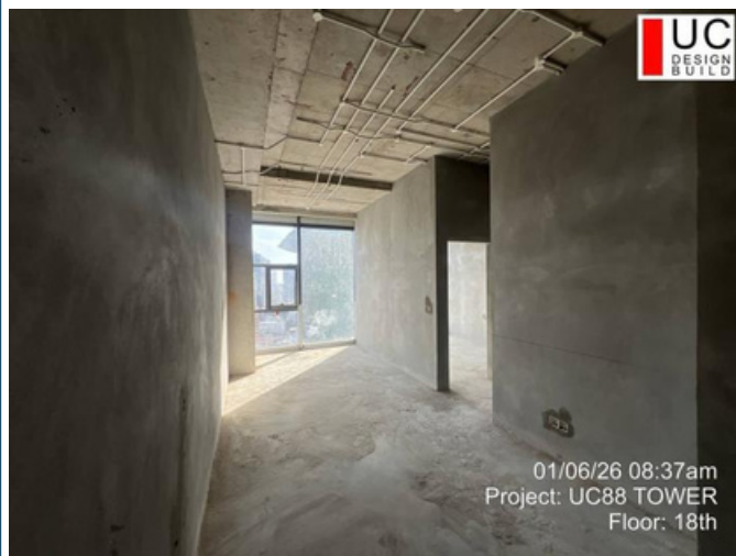
Floor: 18F Date: 06-Jan-2026 Work: MEP work
