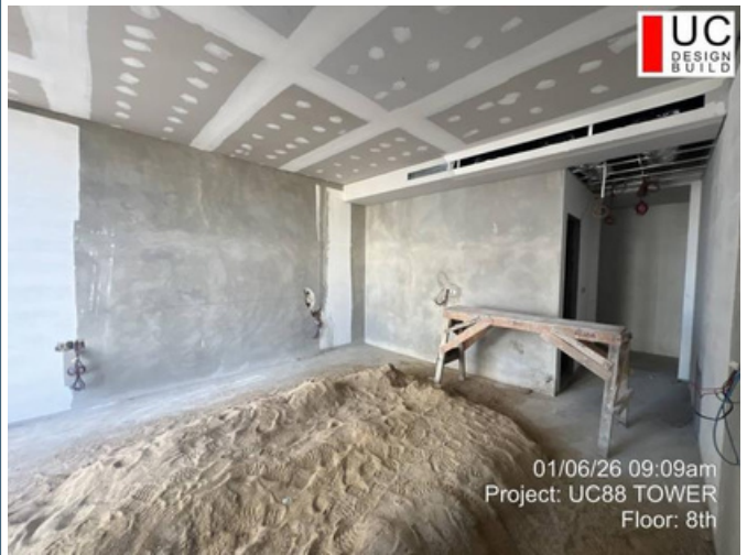
Floor: 8F Date: 06-Jan-2026 Work: Ceiling work
