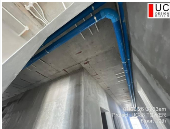
Floor: 19F Date: 06-Jan-2026 Work: MEP work
