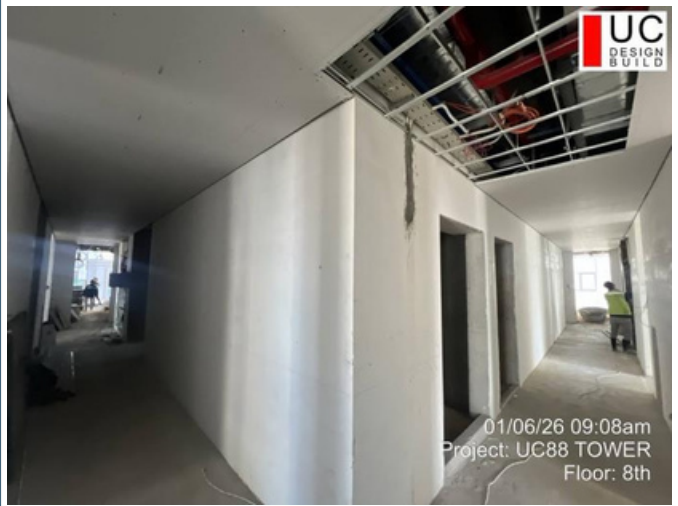
Floor: 8F Date: 06-Jan-2026 Work: Skim coat work
