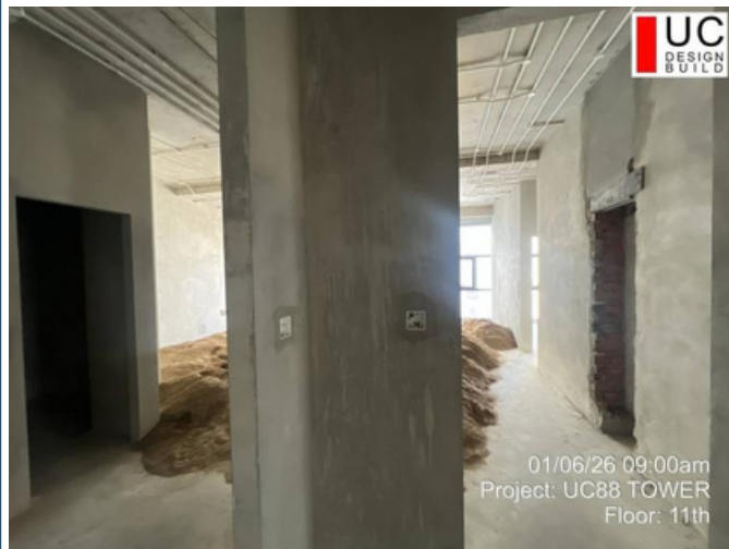
Floor: 11F Date: 06-Jan-2026 Work: Masonry work
