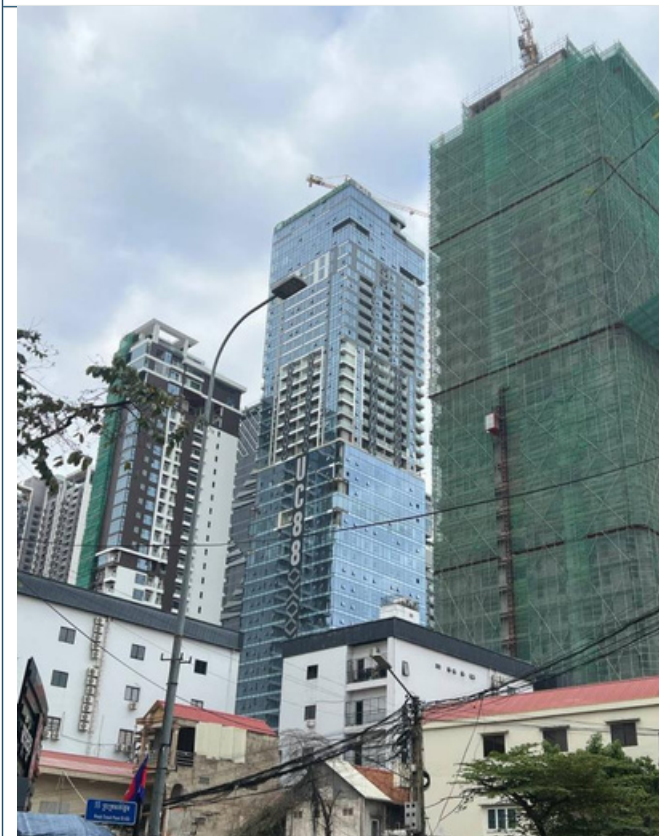
Floor: South View (rear)
