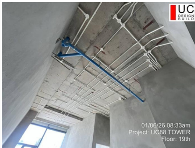
Floor: 19F Date: 06-Jan-2026 Work: MEP work
