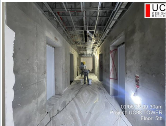
Floor: 5F Date: 06-Jan-2026 Work: Marble work
