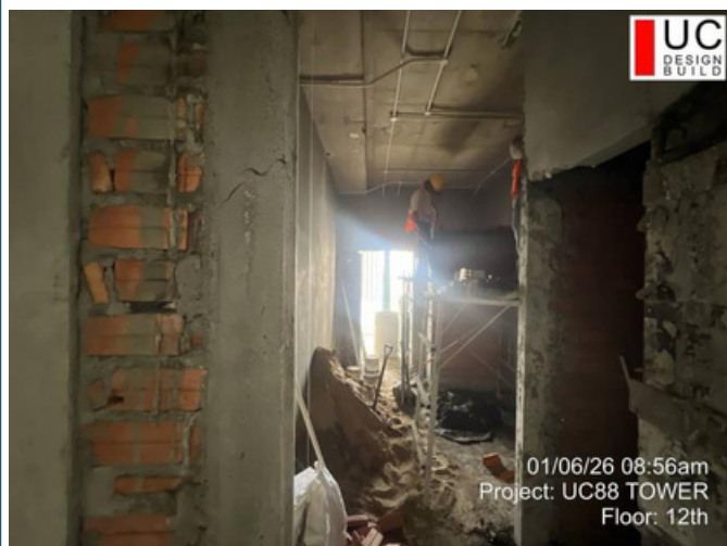
Floor: 12F Date: 06-Jan-2026 Work: Masonry work
