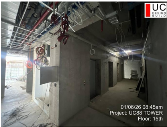
Floor: 15F Date: 06-Jan-2026 Work: MEP work
