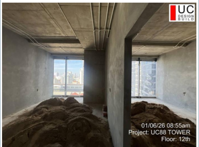
Floor: 12F Date: 06-Jan-2026 Work: Masonry work
