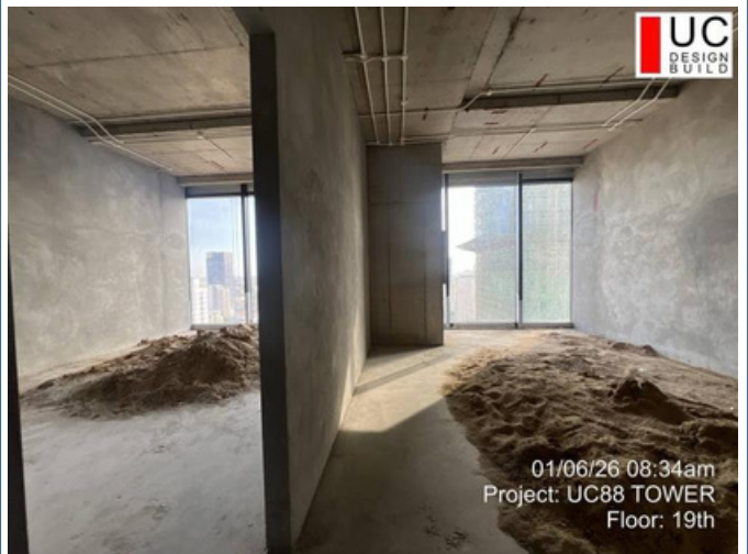
Floor: 19F Date: 06-Jan-2026 Work: Masonry work
