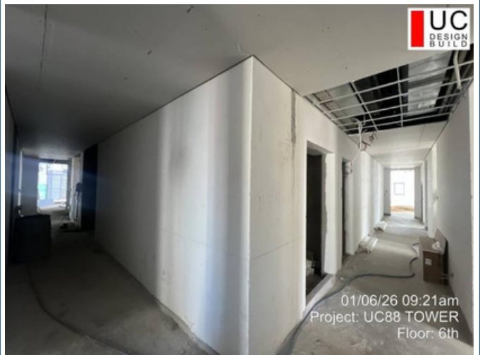
Floor: 6F Date: 06-Jan-2026 Work: Skim coat work
