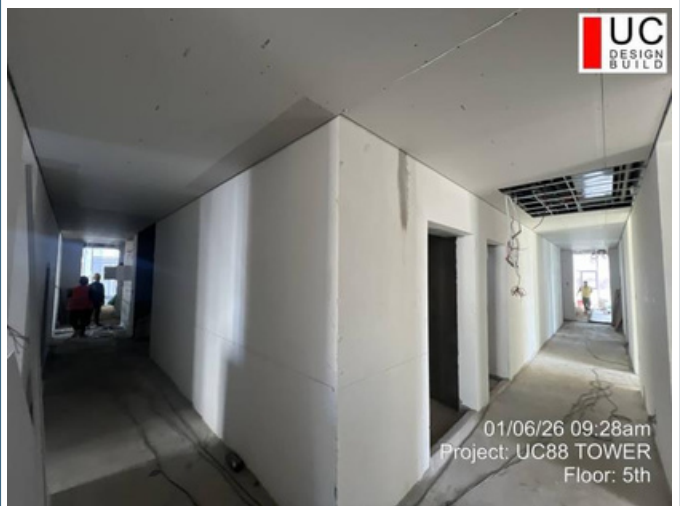
Floor: 5F Date: 06-Jan-2026 Work: Ceiling work
