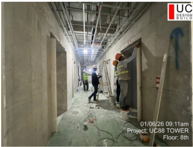
Floor: 8F Date: 06-Jan-2026 Work: Marble work
