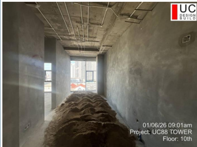
Floor: 10F Date: 06-Jan-2026 Work: MEP work
