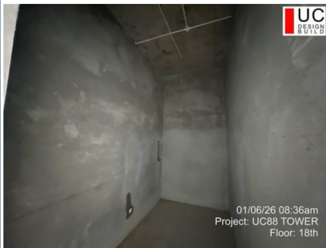
Floor: 18F Date: 06-Jan-2026 Work: MEP work
