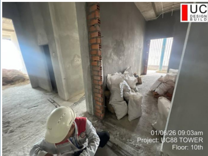
Floor: 10F Date: 06-Jan-2026 Work: Masonry work
