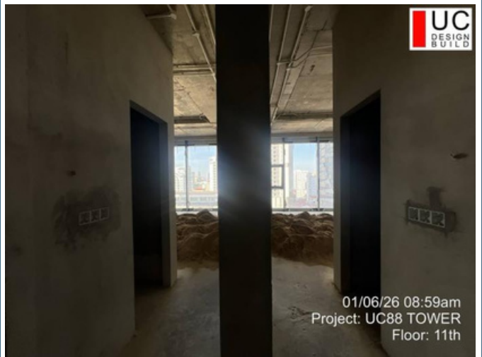
Floor: 11F Date: 06-Jan-2026 Work: MEP work
