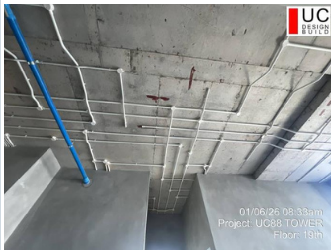
Floor: 19F Date: 06-Jan-2026 Work: MEP work
