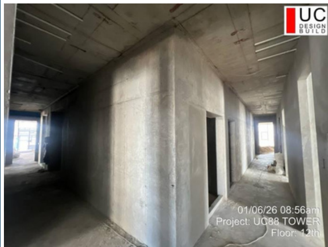
Floor: 12F Date: 06-Jan-2026 Work: MEP work
