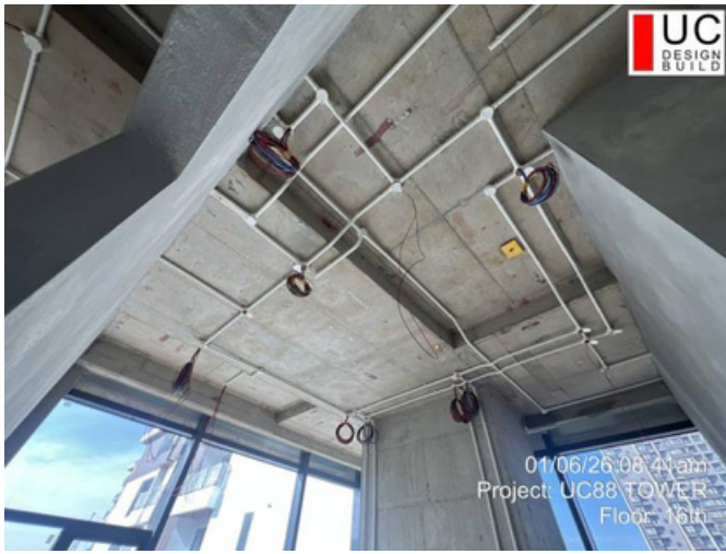
Floor: 16F Date: 06-Jan-2026 Work: MEP work
