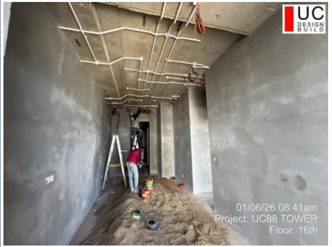
Floor: 16F Date: 06-Jan-2026 Work: MEP work
