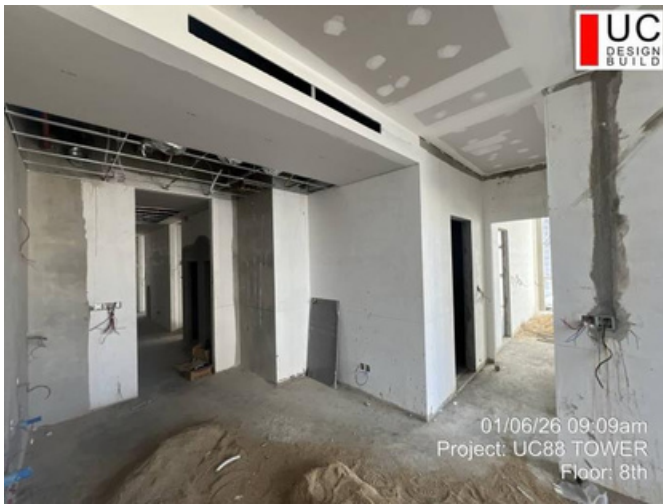
Floor: 8F Date: 06-Jan-2026 Work: Ceiling work
