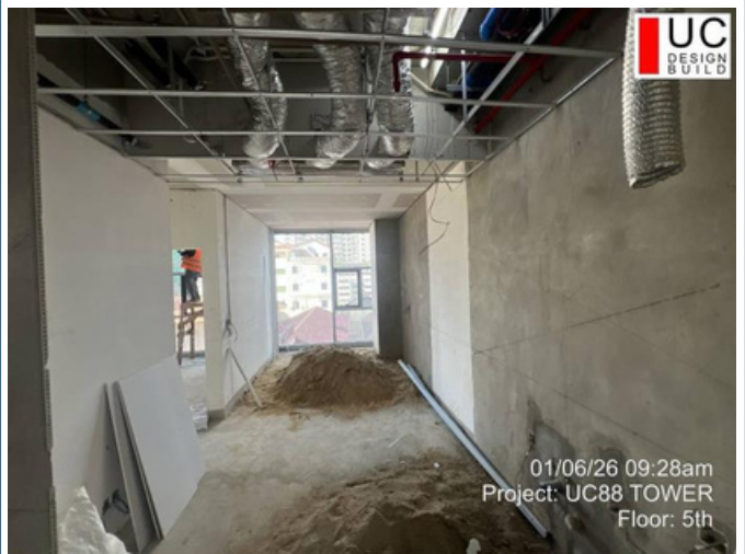
Floor: 5F Date: 06-Jan-2026 Work: Ceiling work
