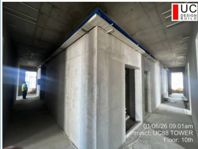
Floor: 10F Date: 06-Jan-2026 Work: MEP work
