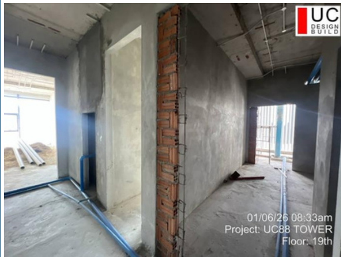
Floor: 19F Date: 06-Jan-2026 Work: Masonry work
