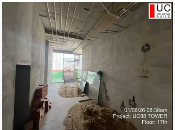
01/06/26 08:38am Project: UC88 TOWER Floor: 17th
