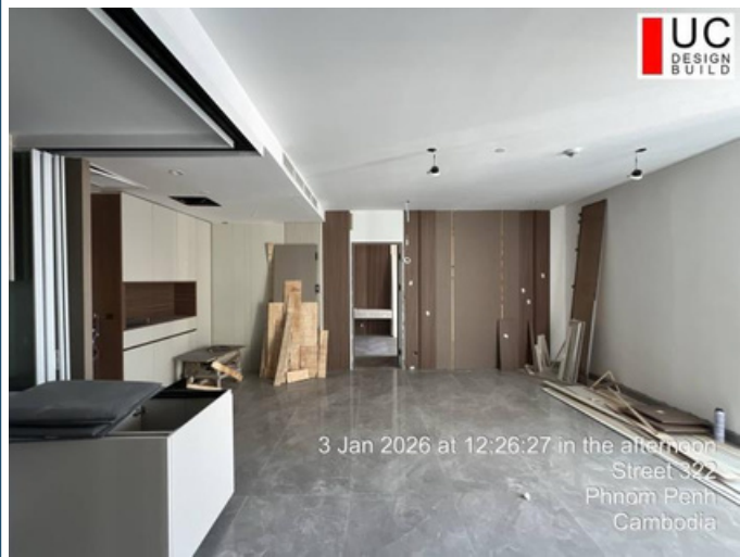
Floor: 33F Date: 03-Jan-2026 Work: Built in Work
