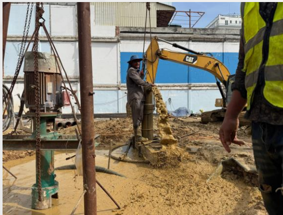
Cleaning pile using airlift.
