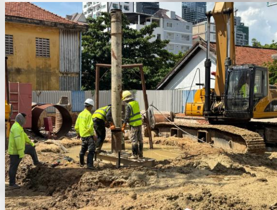
Inserting trimie pipe.
